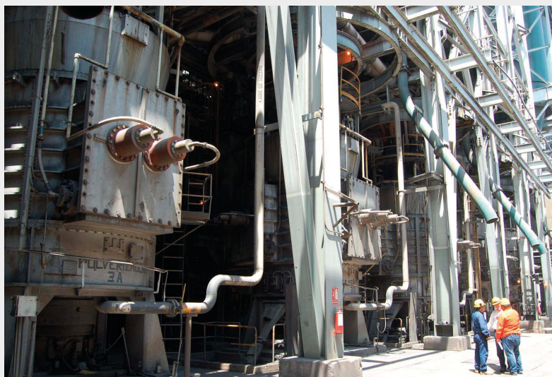
RKB technical on-field activity in a power plant
